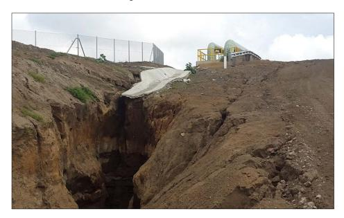
FIGURE 3: A deep crevasse caused by flash floods due to the loose cover of the pyroclastic material. The steam line and fence will be washed away if no remedial measures are taken.
