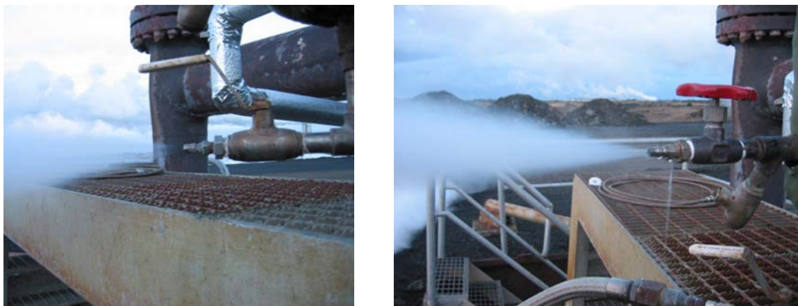
FIGURE 4: Steam sampling outlet on a Webre separator releasing a dry vapor (left) and a mixture of liquid and vapor (right).
