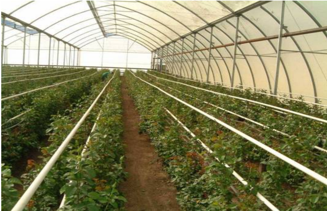
FIGURE 2: Oserian greenhouse heating using geothermal energy
