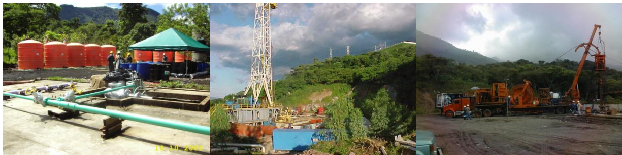
FIGURE 1: a) Chemical injection through well head, b) Chemical injection with a drill rig and c) Chemical injection with a coil tubing.
