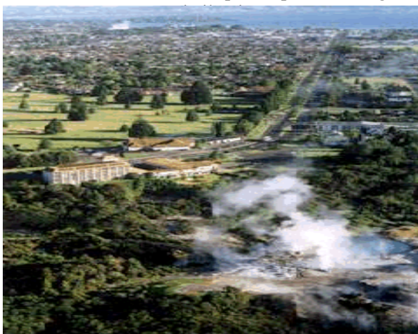
FIGURE 7: Geothermal power plant at Rotorua, Newzealand.
