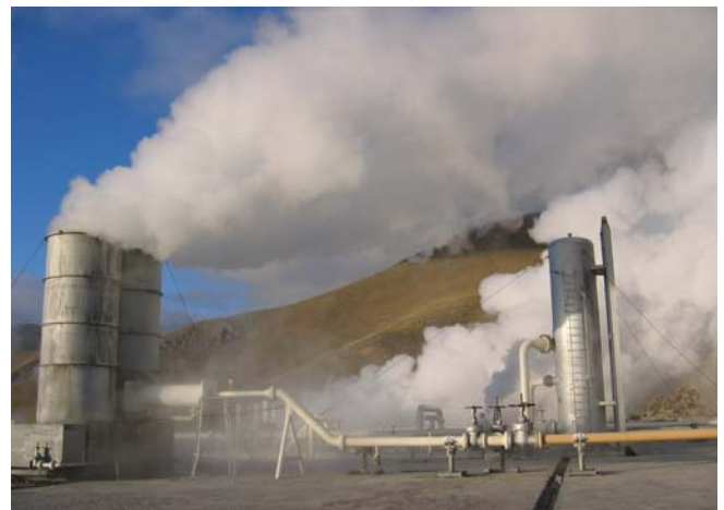
Figure 4. Discharge test (well NWS-4)
