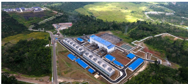
FIGURE 2: Ulubelu geothermal power plant units 3 and 4 (PGE, 2019)
