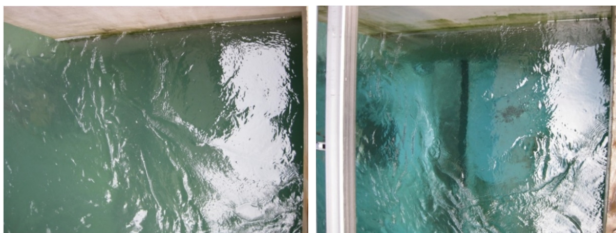
FIGURE 13: Left: Cooling water in the Olkaria II basin during dosing; Right: When no dosing is taking place (SKM, 2011)
