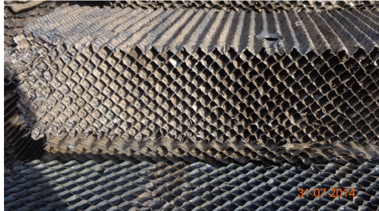
FIGURE 15: Cooling tower fills removed during unit 1 overhaul maintenance in July 2014
