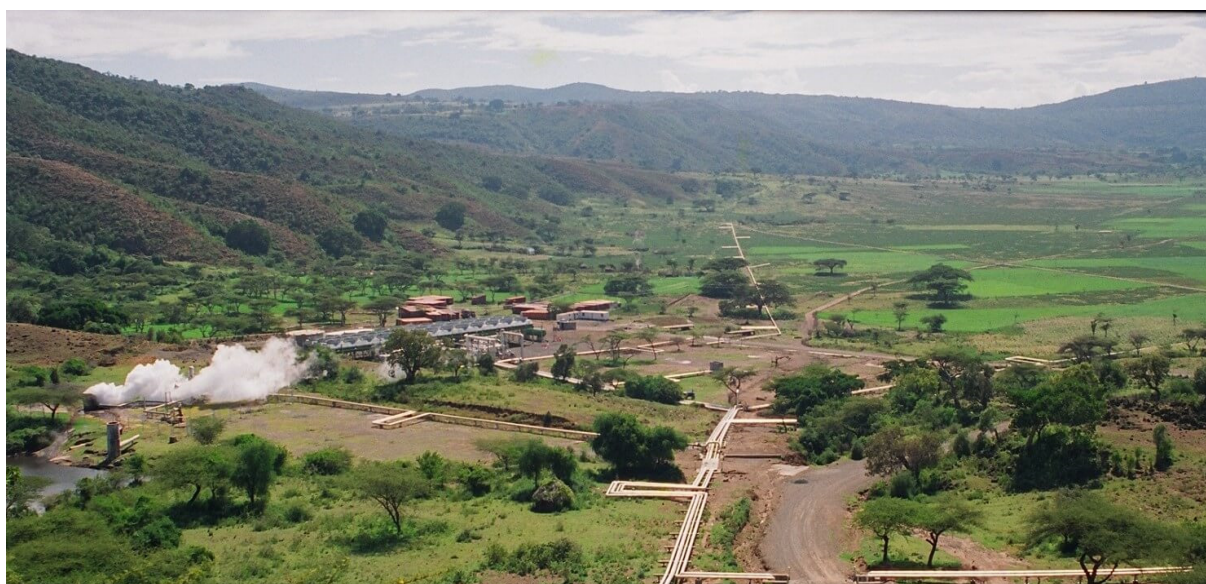
FIGURE 4: Aluto geothermal power plant site (courtesy of Reykjavik Geothermal)
