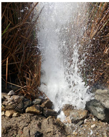
FIGURE 2: Burst fresh water supply line
