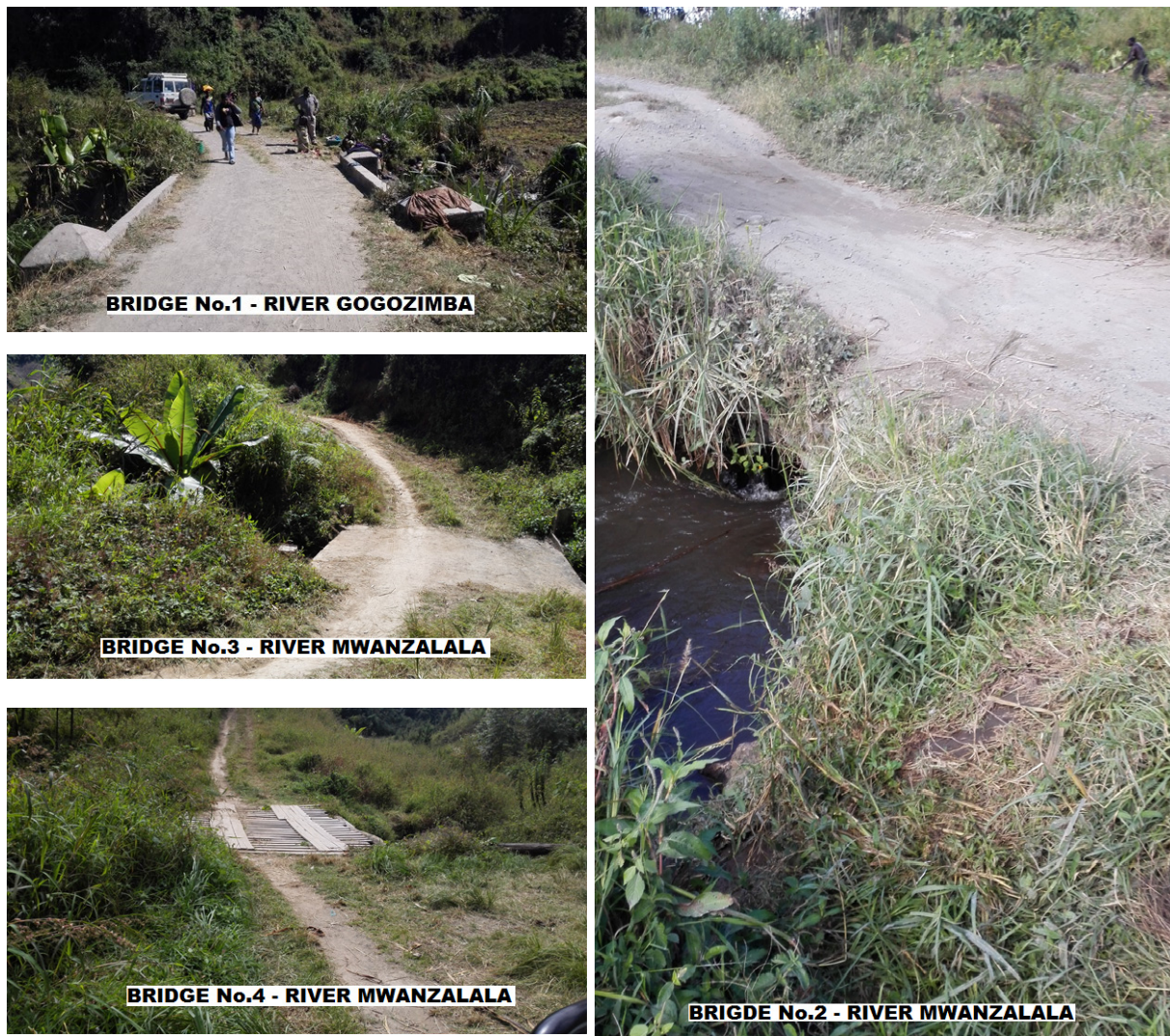
FIGURE 8: Existing bridges toward drill site NB-2 (Field Study, June 2016)
