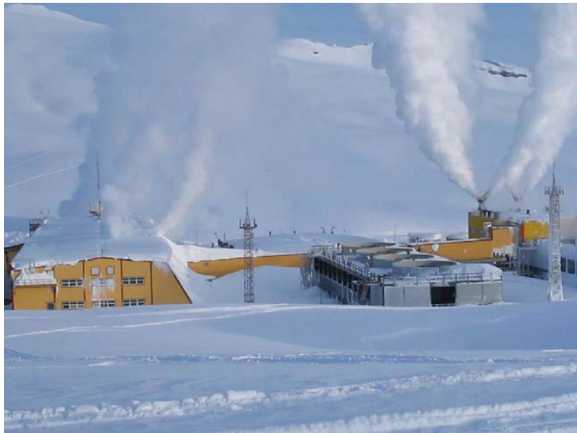
FIGURE 2: Outward appearance of Mutnovsky geothermal power plant
