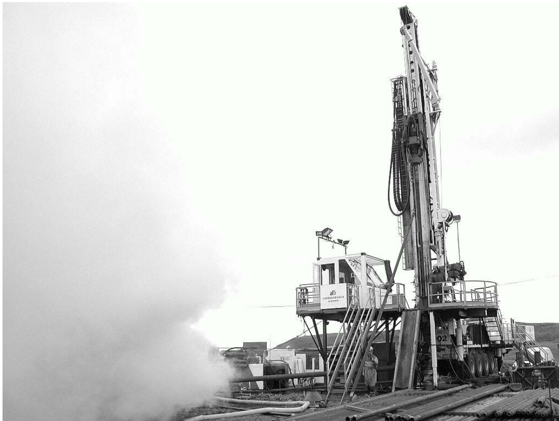
Figure 9: Well being reamed of calcite scale with the well flowing.
