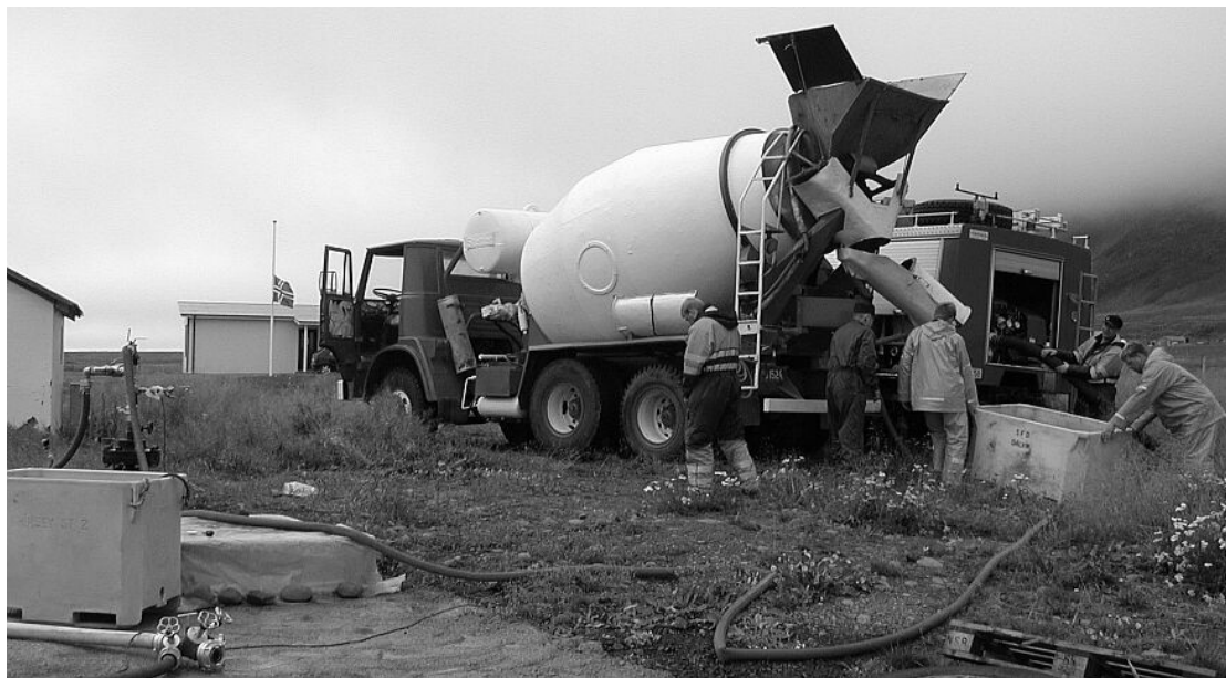
Figure 7: A well being killed with 1.2 \text{ g/cm}^3 brine mixed in a ready mix truck and then pumped with a fire engine. Two mixes were enough to kill the well with artesian pressure of 3.6 bar-g.
