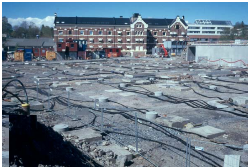
Figure 16: BHE-field in Nydalen, Oslo, Norway, before completion of the buildings (May 2003).
