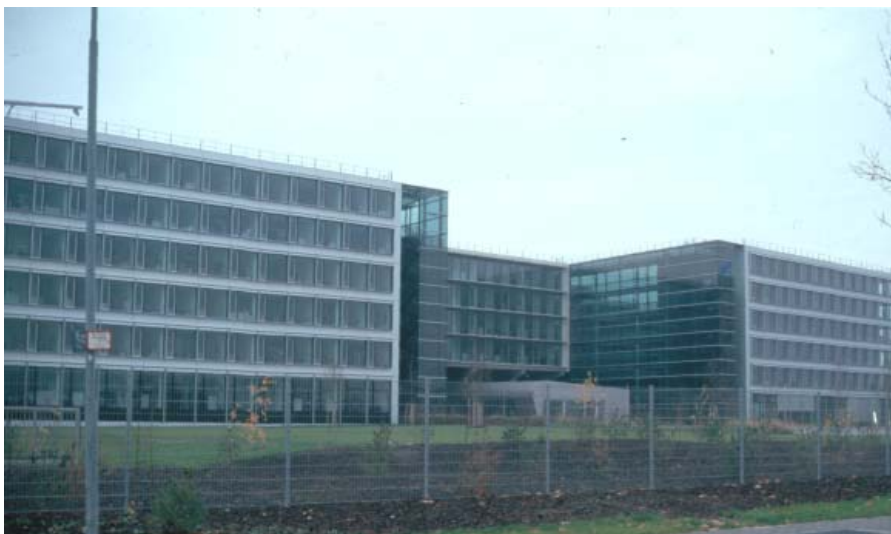
Figure 14: New headquarters of DFS, heated and cooled by GSHP.
