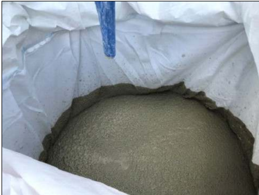
Figure 3. Concrete waste water filtration system
