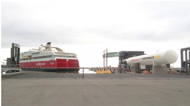
Figure 2 LNG bunkering station in Hirtshals
