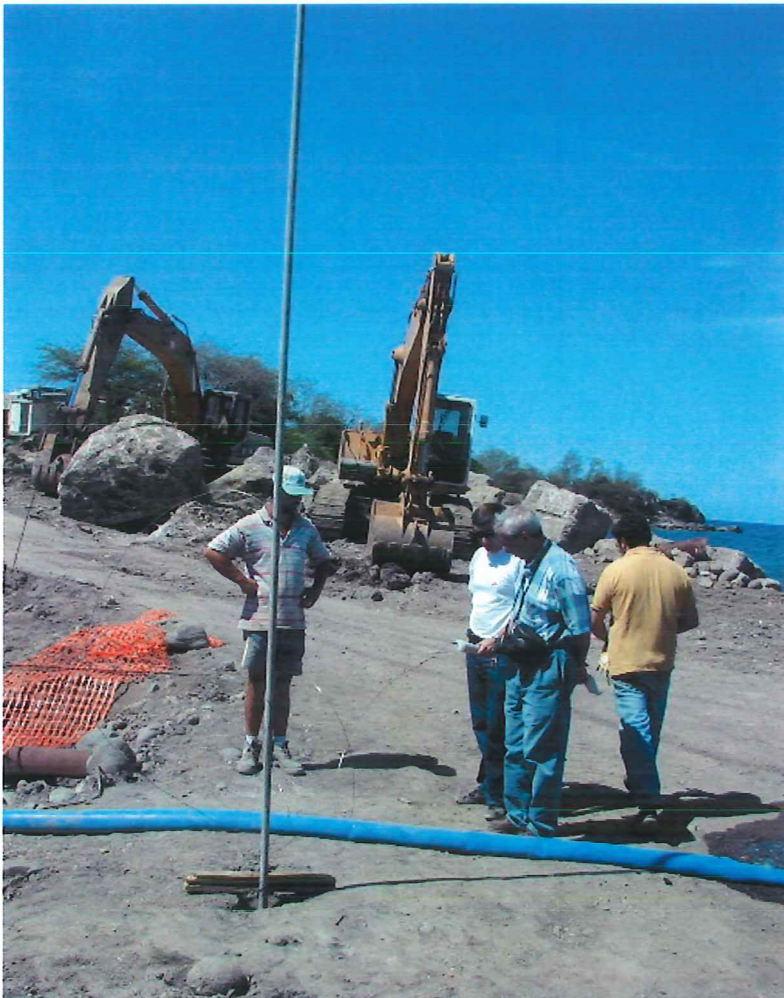
Photo 14. An encapsulated thermocouple wire strapped to a pipe finally worked.
