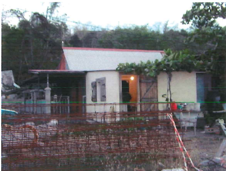
Photo 4. Another house next to photo 3 with a warm floor. The living room floor in the top left corner of the house measured 46°C. Other parts of the floor were warm as well.
