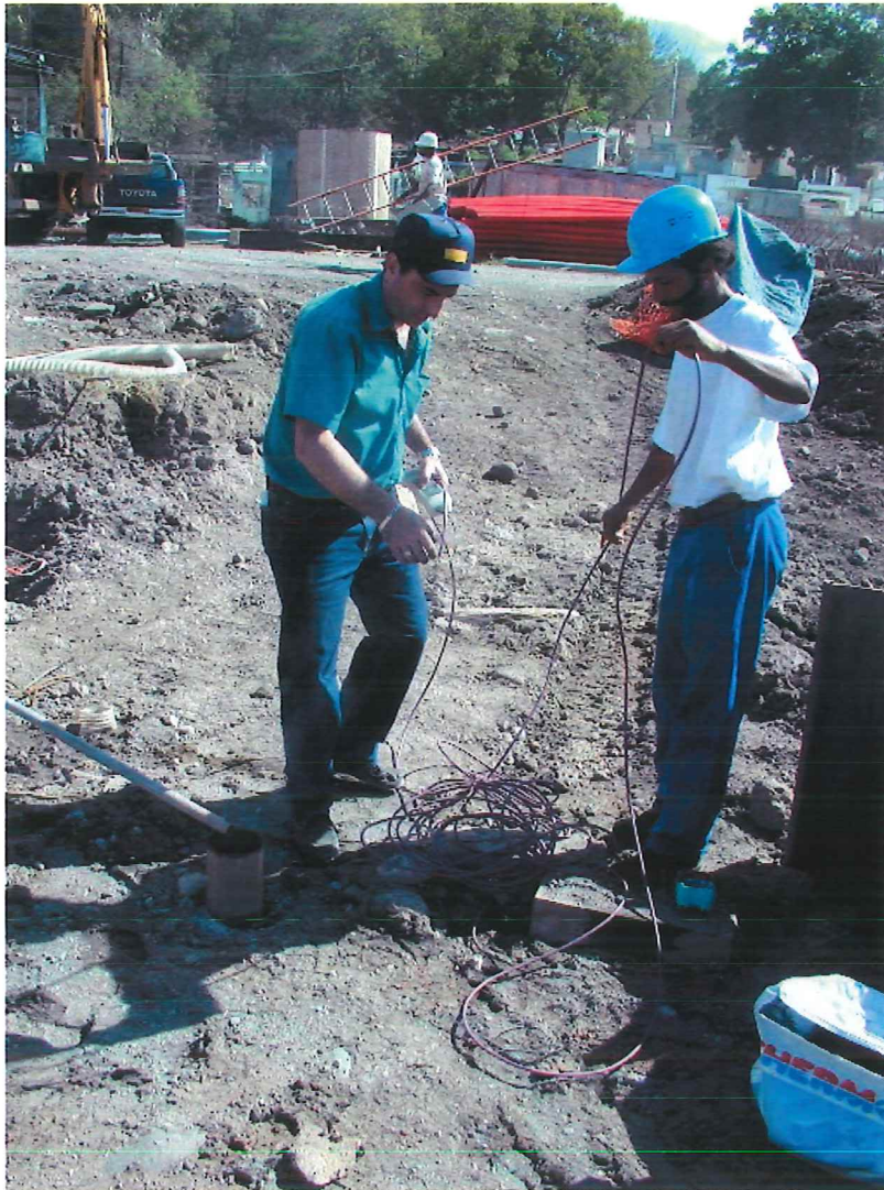
Photo 11. Logging of the observation hole with a thermocouple. The wire insulation failed due to poor temperature resistance of the plastic isolation tape.
