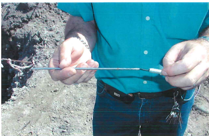
Photo 12. Close-up of failure of thermocouple wire.
