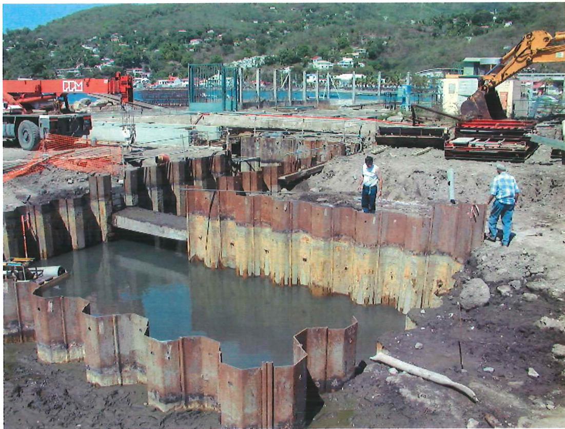
Photo 16. Photograph of the pit Saturday 15.03.2003 after being drained by pumping. There was no increase in thermal activity during this period. Only a few gas bubbles were surfacing near the pump barge.
