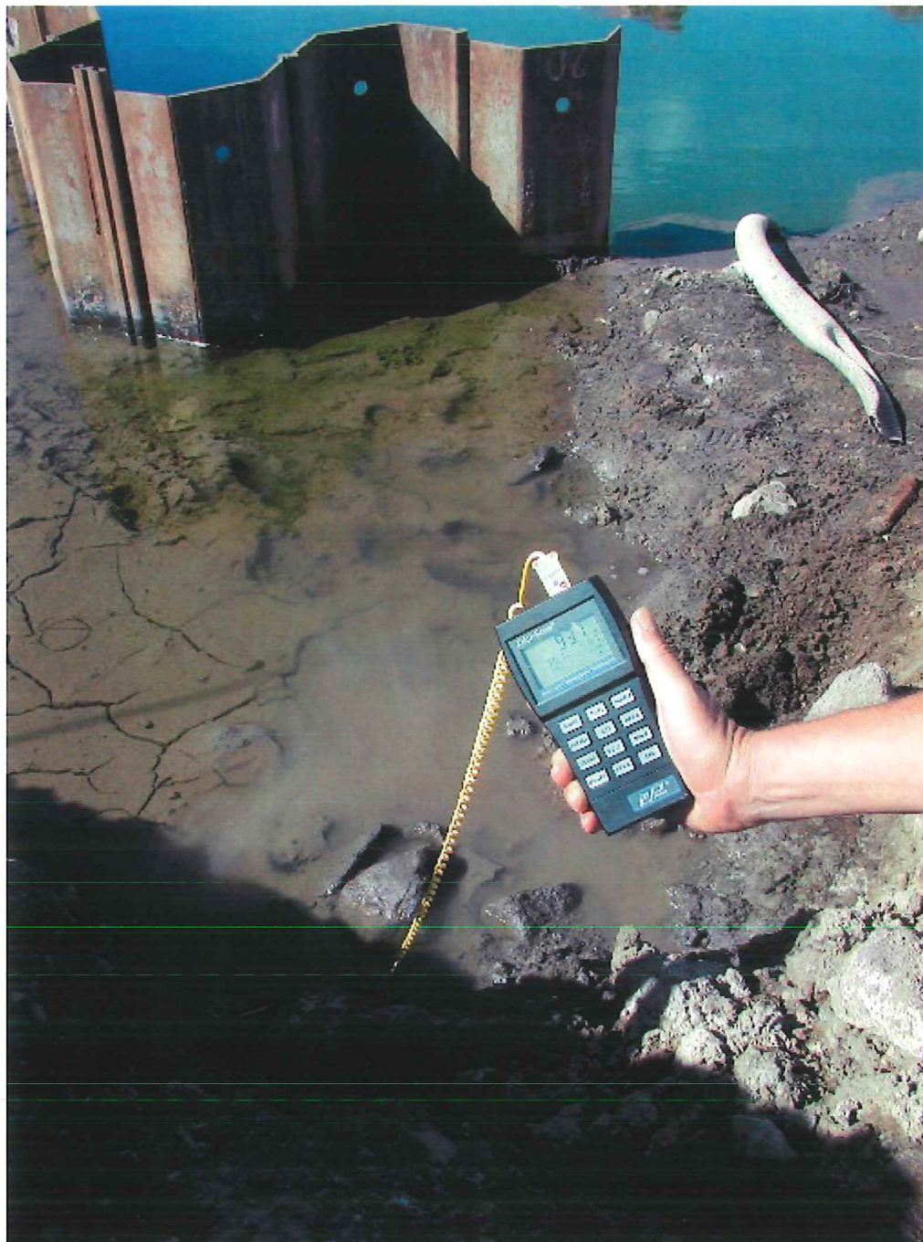
Photo 7. Hot mud (93,1°C) on surface just outside the steel piles. The mud is very soft and did not support the authors weight.
