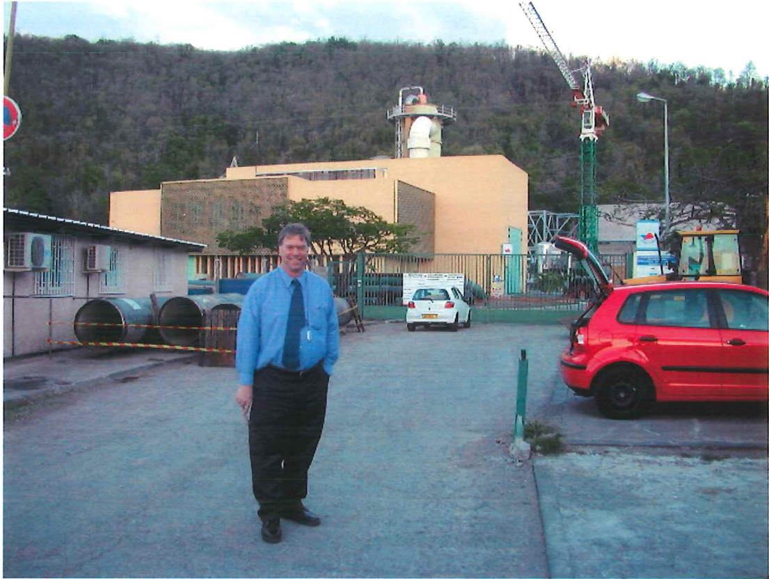
Photo 1. Sverrir Thorhallson (report author) in front of the Bouillante power plant. Recently removed sea water pipeline in background.
