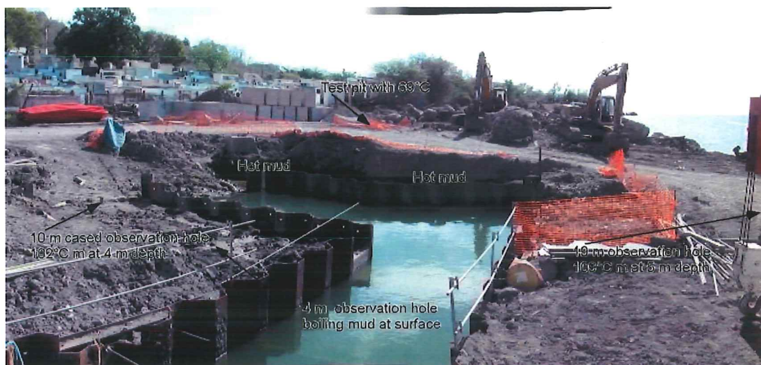
Photo 8. Photograph of pit showing position of hot spots and three observation holes.
